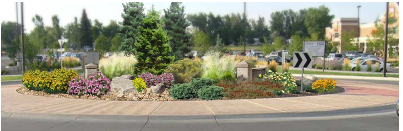
Illustrations of roundabout landscaping approach with mixed planting, boulders, mulch and hardscape patterns all designed in conjunction. Lower graphic shows the inclusion of landscape walls.
