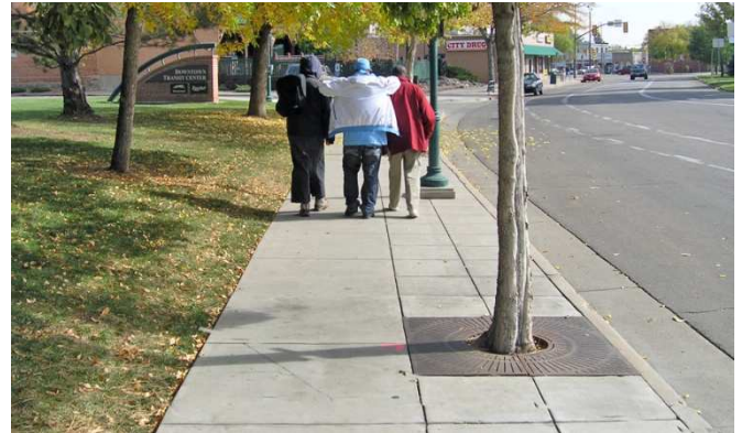
8-foot sidewalk with 4'x4' tree grates, where there is an abutting landscape area.
