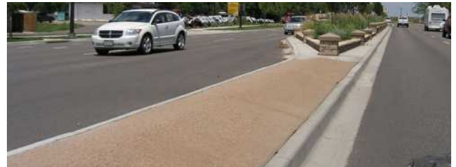
Tan exposed-aggregate concrete median paving.
