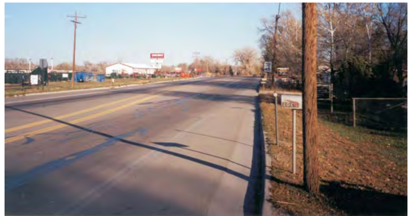
7. View along US 287 east
