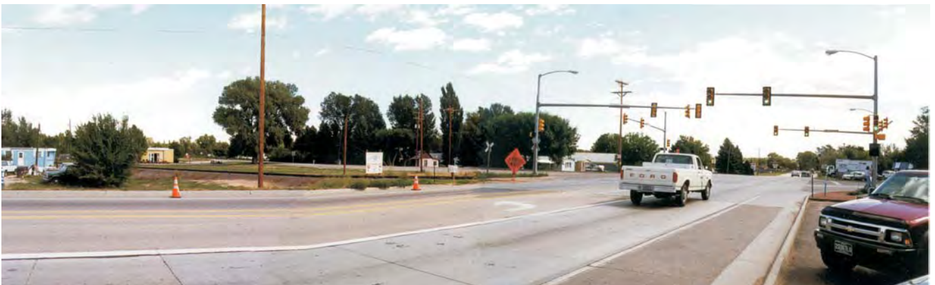
8. View northeast along US 287 toward intersection of North Shields Street and Union Pacific RR crossing
