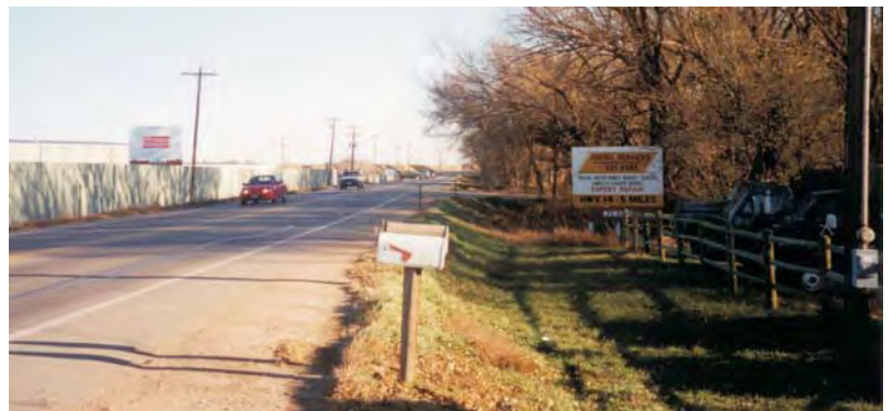
4. View east along US 287 near Terry Lake Dam
